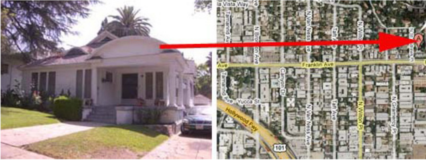
1912 St Andrews- before demolition
