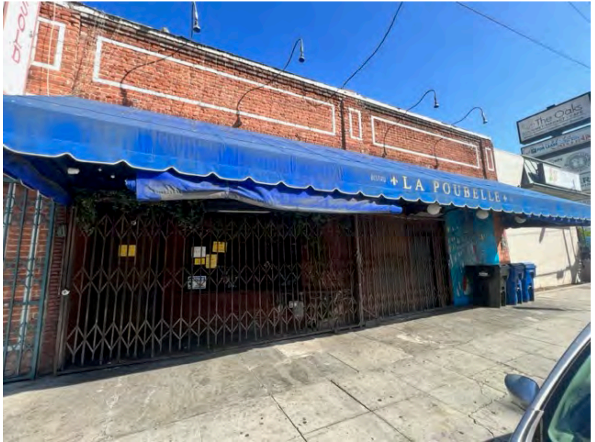
Franklin Ave., entryway. Direction: Northeast
